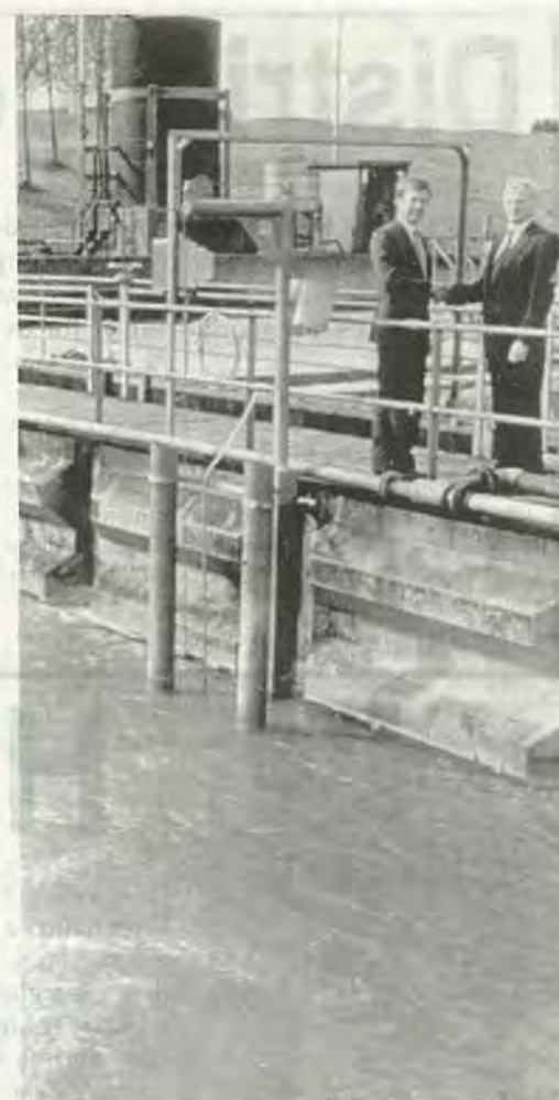
An effluent tank at Bass Brewing, Runcorn, where a Venturi aerator is helping reduce smells and save money. UTT's Dr. David Walker (left) is pictured with Bass Effluent Treatment Manager Nick Massey.
